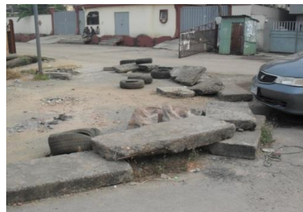
Plate 26. Surulere, Lagos photograph Source: Obiadi's field work (2015). A better photograph of the street, showing the abandoned security gate, gate in disrepair, abandoned tires, concrete slabs, and empty concrete bays at the middle of the road. A van parked at the middle of the road behind the concrete slabs.
