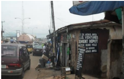
Plate 17. Zik Avenue's commercial area showing a building and electric pole atop the pedestrian sidewalk. Source: Obiadi's field work (2015). The electric pole has nothing, but cut and none functional wires dangling over people's head. The building sitting atop the pedestrian sidewalk is in total disrepair and the little part of the sidewalk left for the pedestrians was covered with empty cartons, shielding off and prevention the designated users' access.
